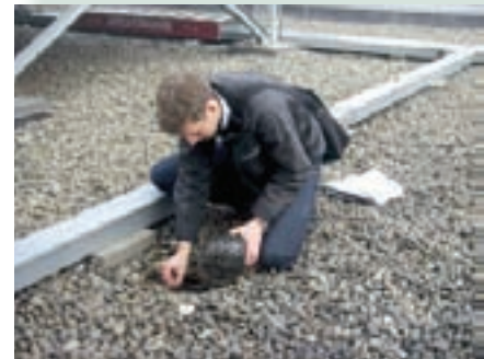
Roof drain cleaning
